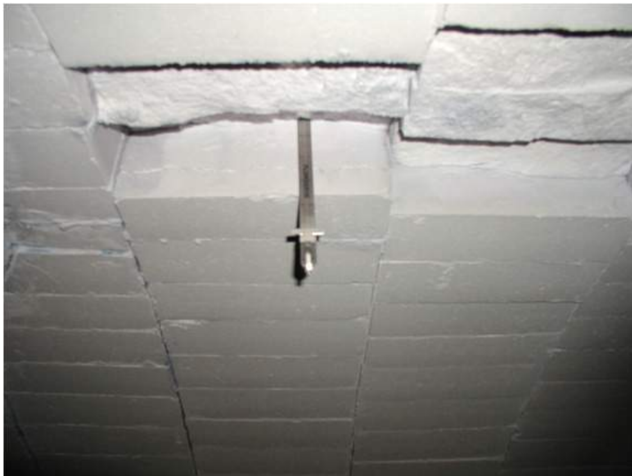
Figure 24—Deteriorated Refractory-tile Lining
