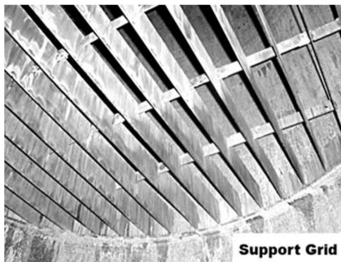
Figure B.54—Support Grid from Below
