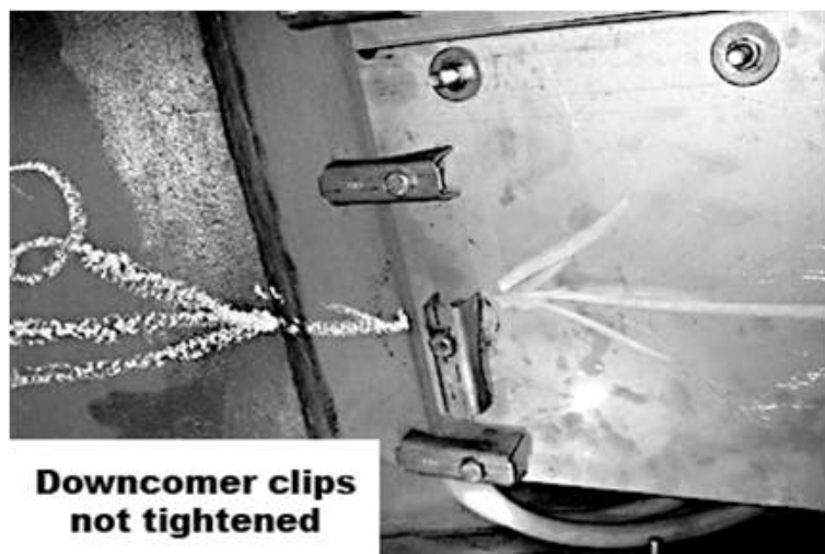
Figure B.88—Downcomer Clamp Loose
