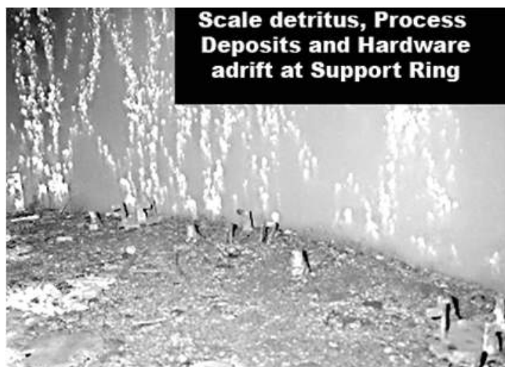
Figure B.90—Deposits Adjacent to Shell are on Ring
