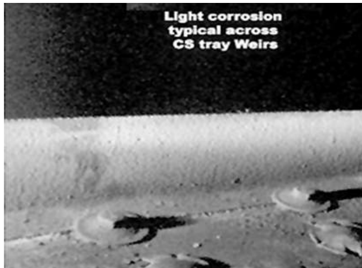
Figure B.85—Light-to-moderate Weir Corrosion
