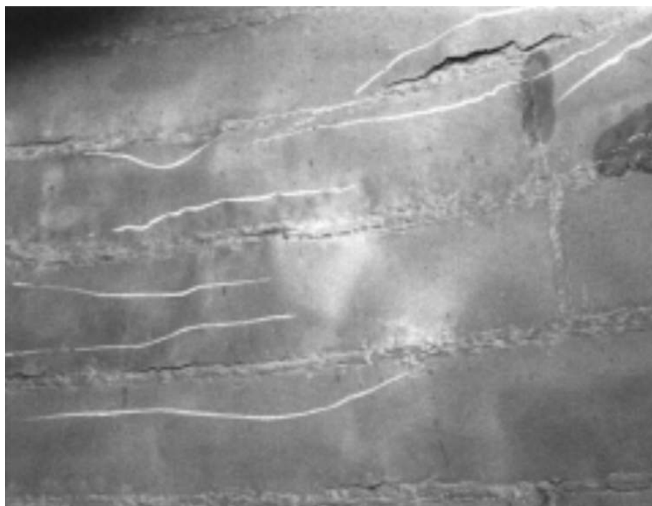
Figure 23—Strip-liner Deterioration
