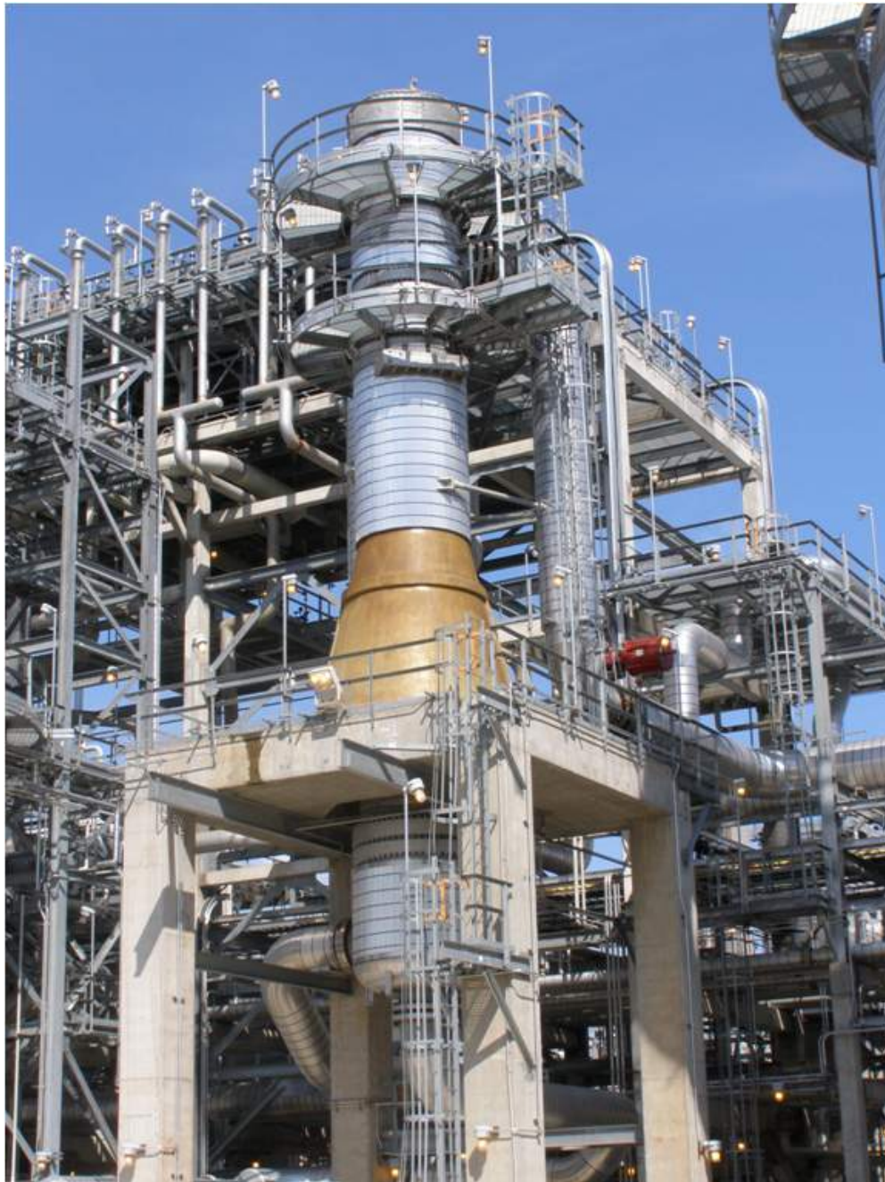
Figure 7—Vertical Heat Exchanger
