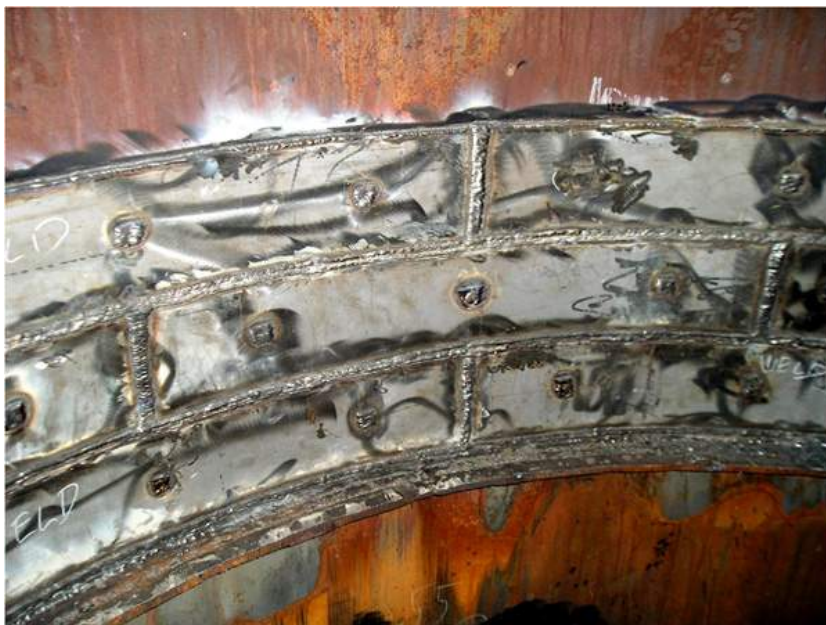
Figure 3—Strip-lined Vessel
