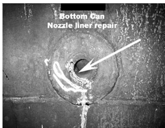
Figure B.59—Stainless Steel Donut Cladding Breech
