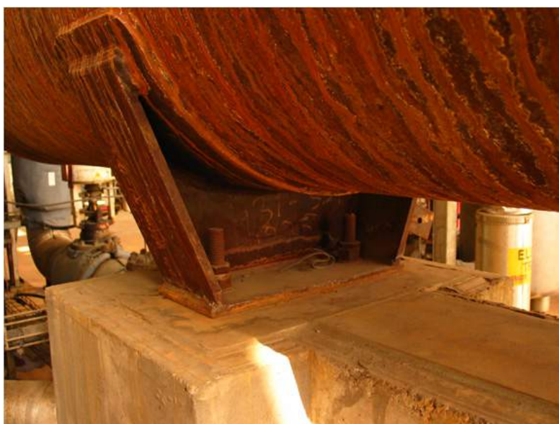
Figure 13—Exchanger Installation and Foundation
