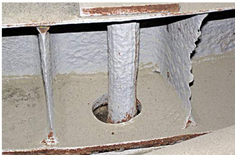
Figure B.25—Corroded Anchor Bolting
