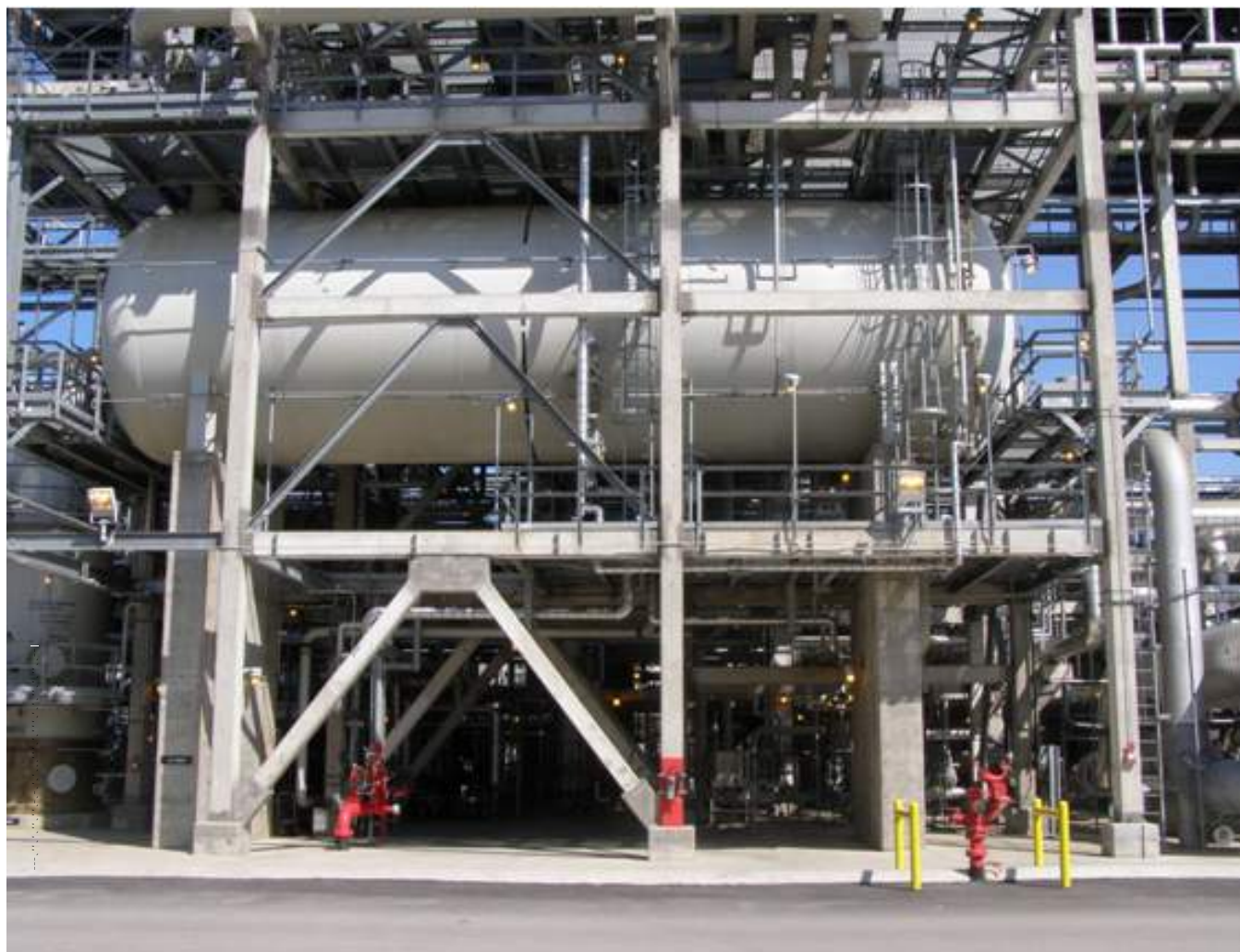
Figure 8—Horizontal Vessel
