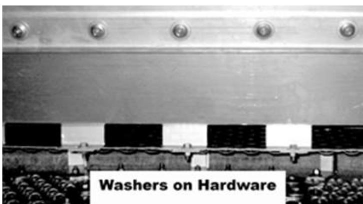
Figure B.49—Hit the Washers, Not the Bolts
