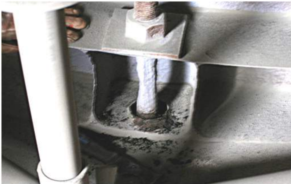
Figure B.26—Corroded Anchor Bolting
