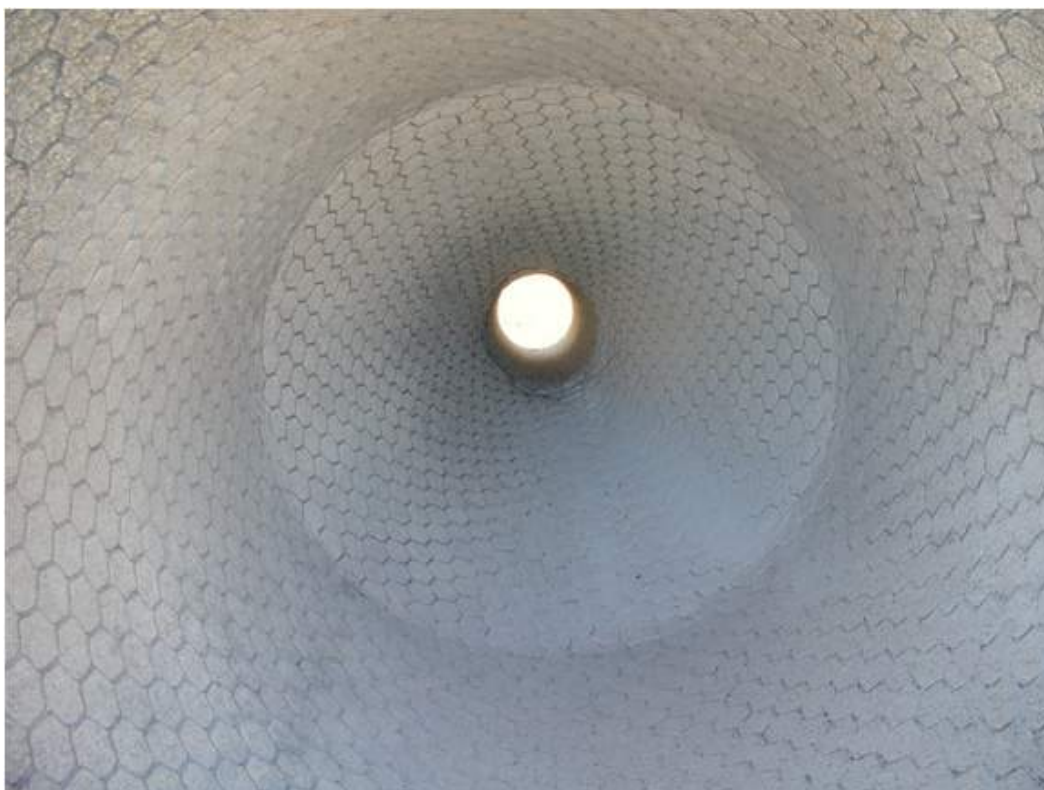
Figure 6—Reinforced Refractory
