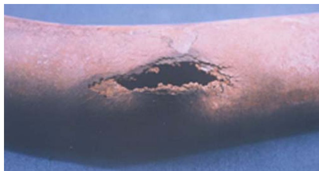
Figure 16—Longer-term Boiler Tube Failure Caused by Poor Circulation and Subsequent Overheating, Oxidation, and Final Failure by Stress Rupture
