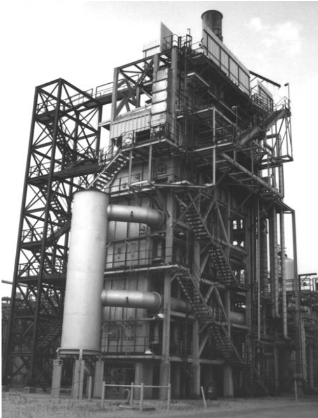
Figure 3—Steam/Methane-reforming Heater
