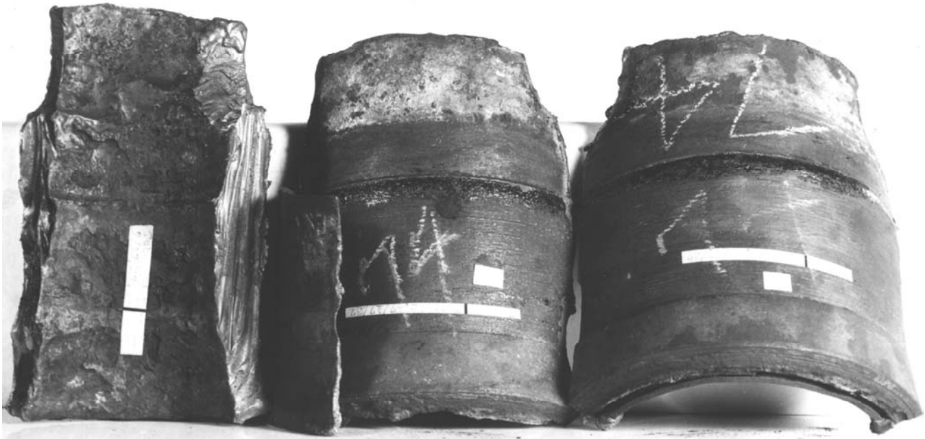
Figure 24—Fitting and Tube that Have Leaked in the Roll
