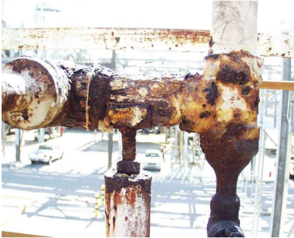
Figure 4-80 – CUI of CS level bridge.
