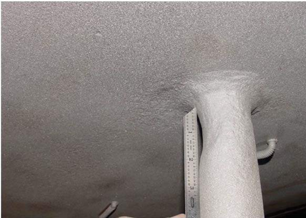
Figure 4-76 – CUI of nozzle on a bottom head.
